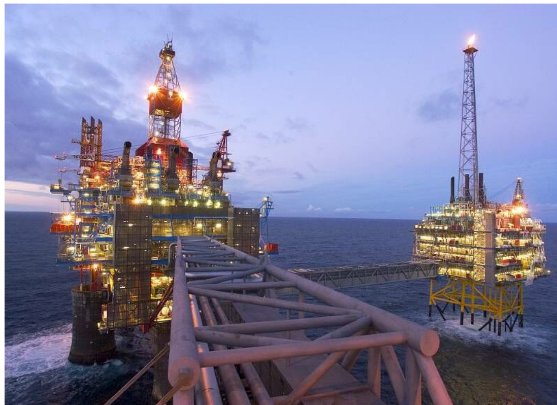
The Sleipner A integrated production, drilling and quarters platform is linked by a bridge to the Sleipner T gas treatment installation
